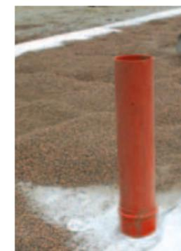
Above-ground section of a vertical inspection pipe,  $d_n$  200 mm
