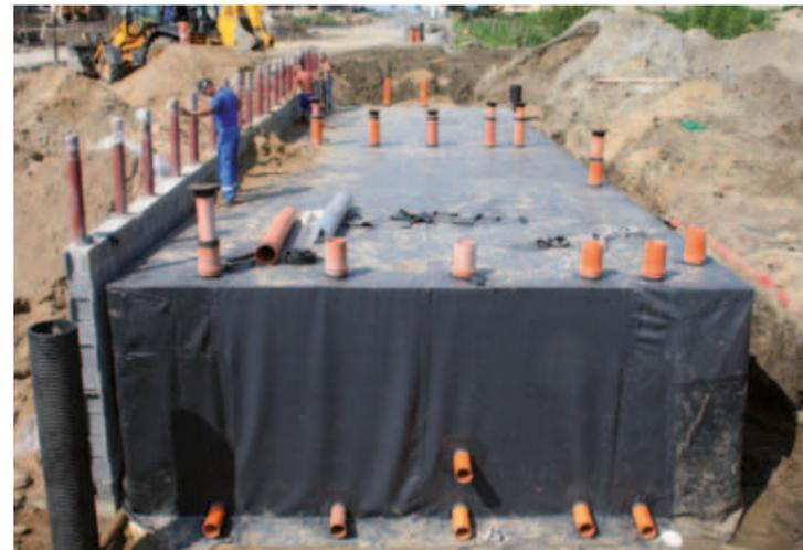
Buffer tank in the rainwater drainage system
