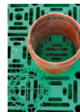
Placing a 200 mm PVC-U pipe in the opening
