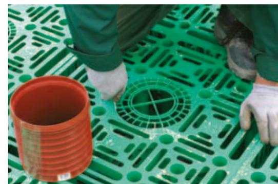
Cutting out the open-work cover of a  $d_n$  200 mm hole located at the top of the box
